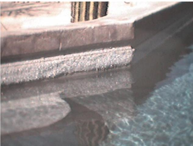
You can see that the tile is almost totally obscured by the deposited crystals, but the grey plaster underwater is not.
